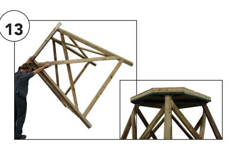
Set the tower stand right side up. Place a level on the braces between each of the legs to determine if the stand needs to be leveled. Wooden shims, or rocks can be used to build up the low sides. Alternately you can use a shovel to dig away soil under the stand foot that needs to be lowered.
