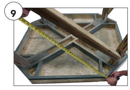
Measure from corner to corner as shown to make sure your leg structure is not twisted before finishing your angle brace attachment.
