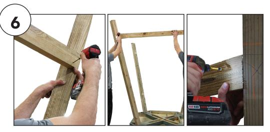
Attach the leg braces with the included screws—lining them up with your 12" mark as shown. (pro tip: start your screws in the braces so that you don't need to fumble with the screws when holding the brace into position).
