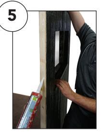
Apply caulk to the side of panel 1 before attaching to panel 2.
