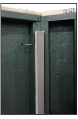
Apply the caulk to the side of panel 2 and add panel 3 to panel 2 making sure they are flush before using screws to permanently attach them together. Continue with all the panels except the last two.
