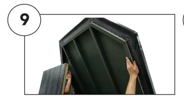
Lift the roof on to the top of the unit and balance on top of the remaining panels. this step requires two people.
