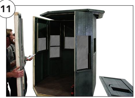
Add the remaining two panels. Remember to use caulk before using screws to secure the panels on the sides and bottoms.
