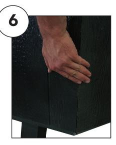
Match up panel 1 and 2 to be sure they are flush before you screw the panels together and before attaching panel 2 to the base.
